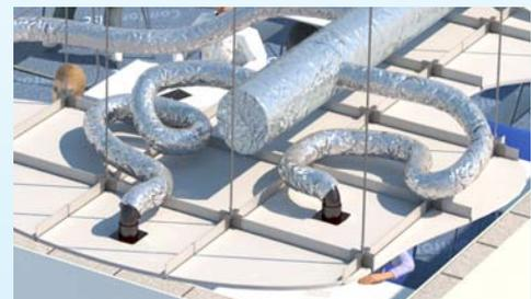
Flexible sound attenuated tubing delivers air to outlets.
