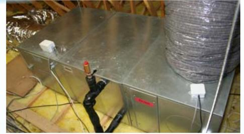
ComfortDisc (3 modules) shown in horizontal configuration in attic.
