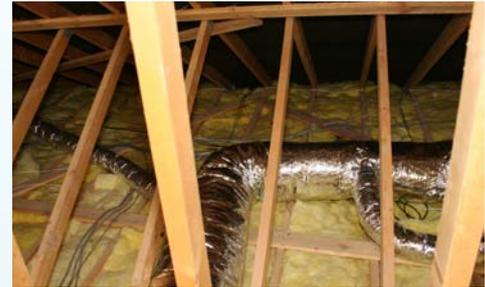
Main Ducting (250mm) and sound attenuated flex tubing in attic.
